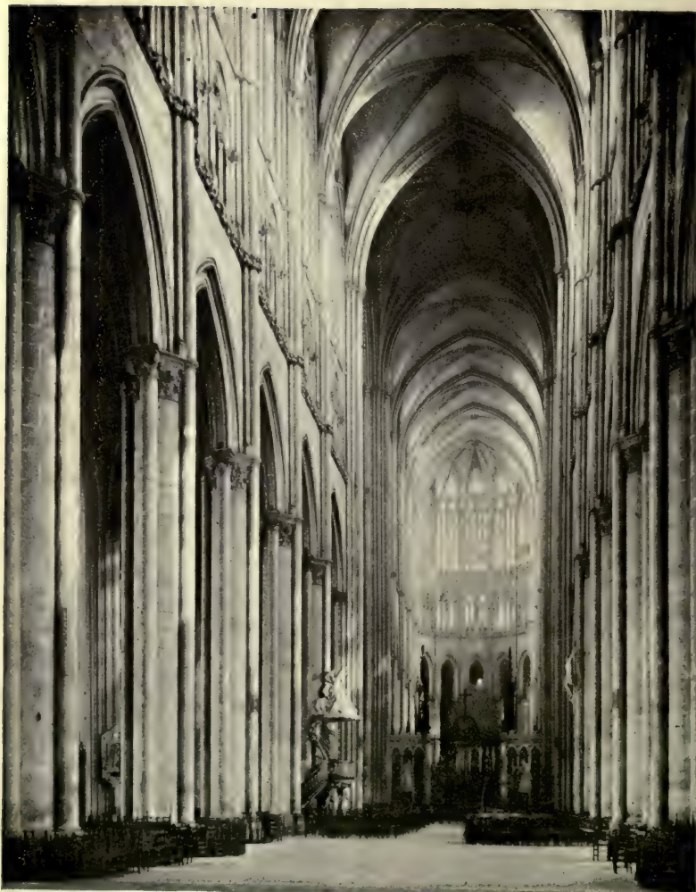
NAVE, LOOKING EAST Cathedral, Amiens
